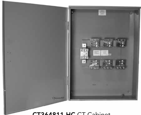
CT364811-HC CT Cabinet and K4722 CT Rack
