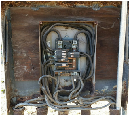
Rusted and outdated unit powering lighting on the Route 250 highway bridge in Sandusky, Ohio.
