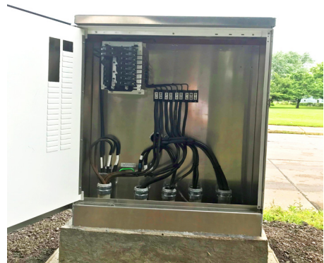
Newly installed unit powering lighting on the Route 250 highway bridge in Sandusky, Ohio.
