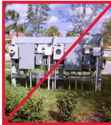
Strut and backboard
