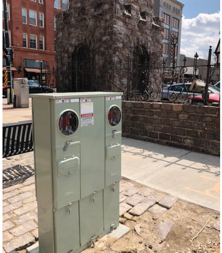
K6342 installation in downtown Milwaukee.
